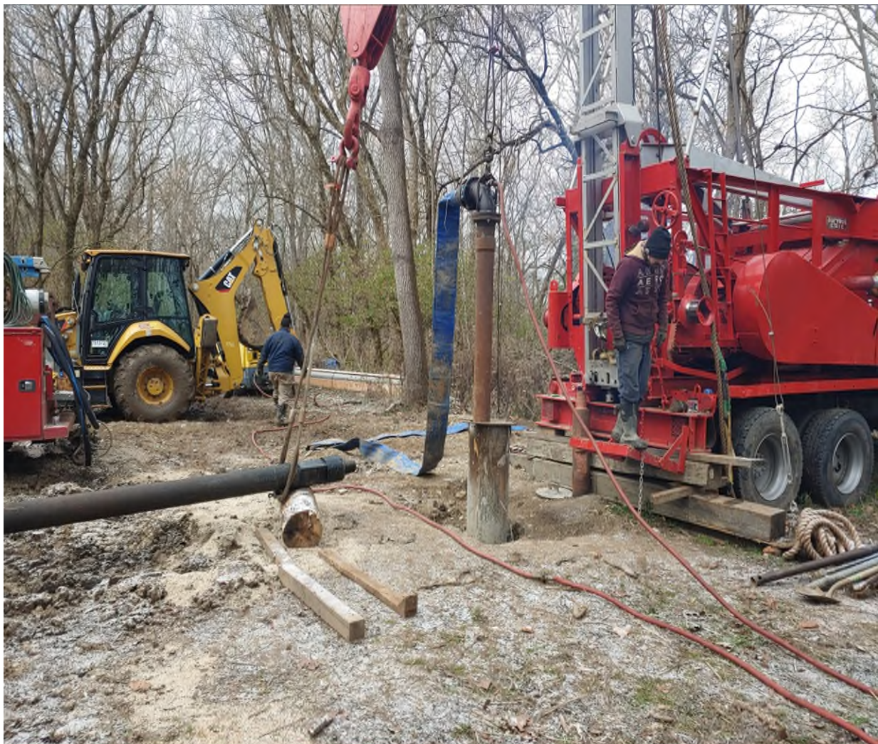
Figure 8. Well development of MJ-PW01 during November-December 2024.
