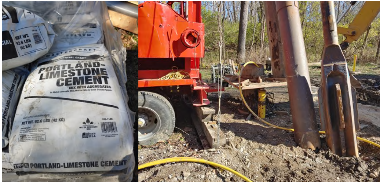
Figure 6. NWS using tremie equipment to seal the annular space of well MJ-PW1 with cement grout, November 26, 2024.
