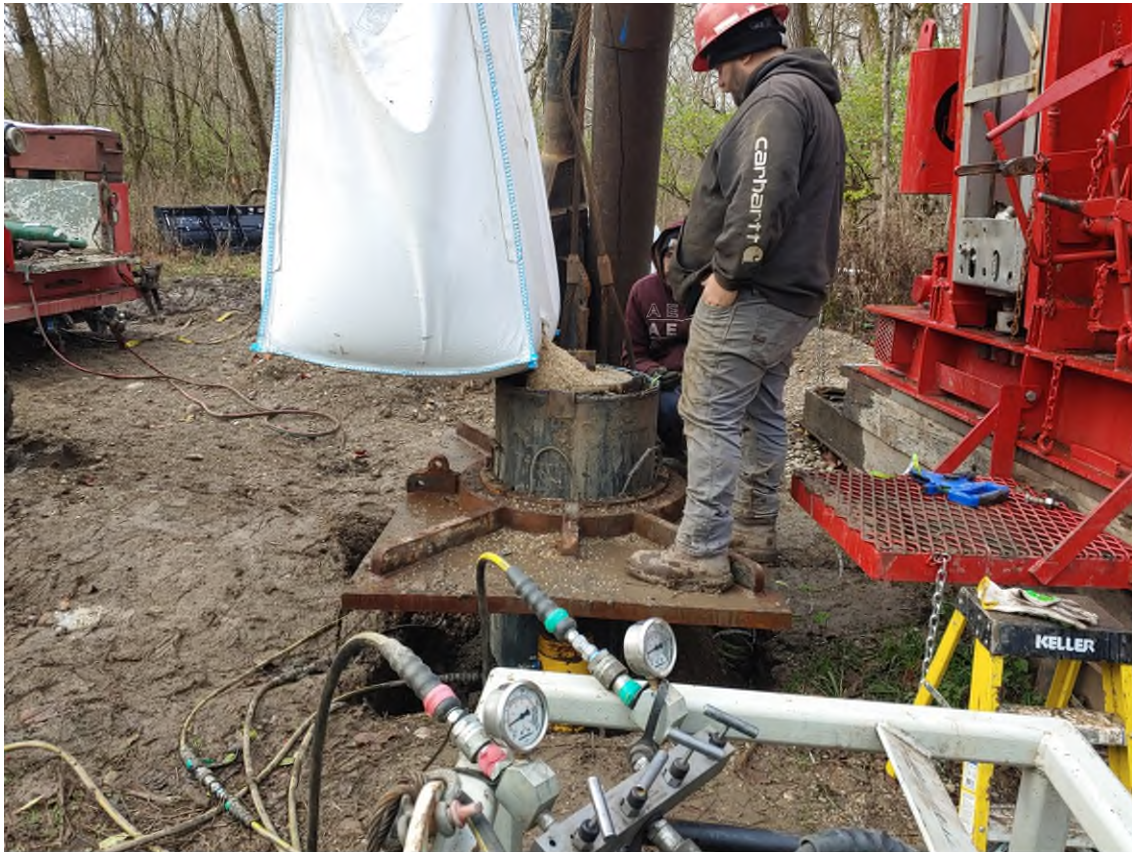
Figure 5. No. 2 Parry sand pack being placed around the well screen, November 22, 2024.
