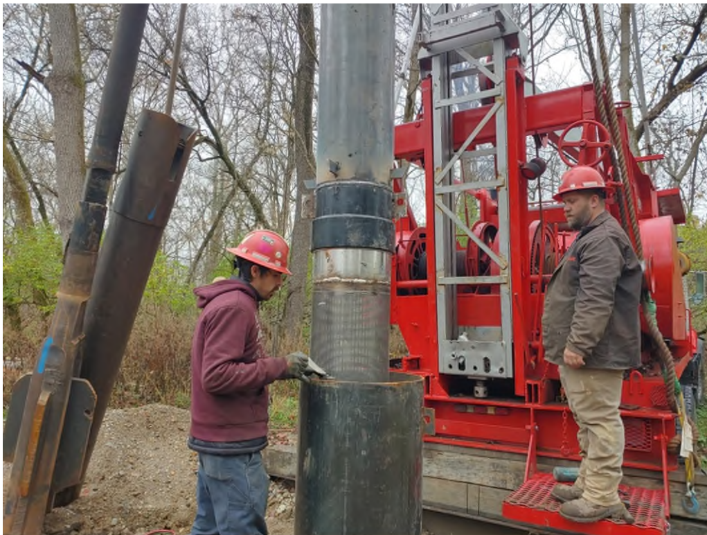
Figure 4. NWS installing MJ-PW1 well screen and casing on November 20, 2024.
