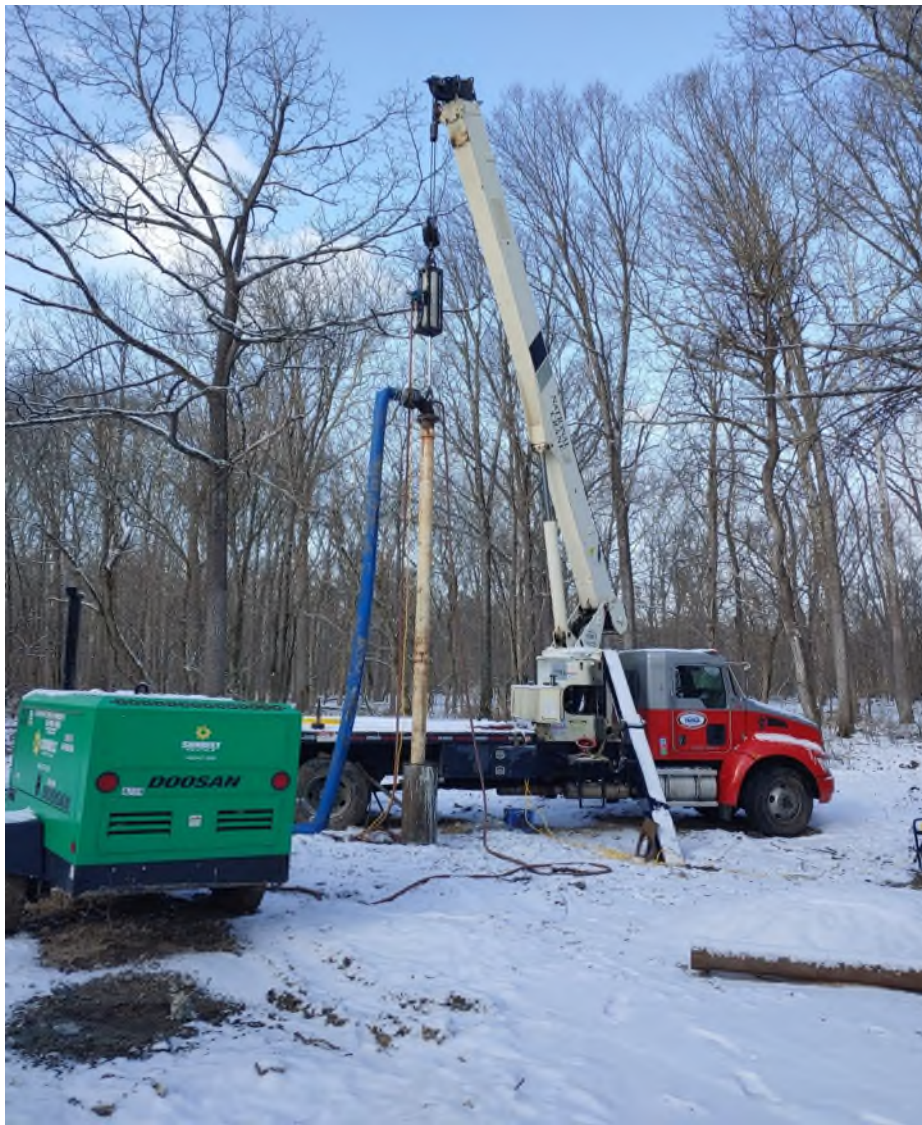
Figure 8. Well development of MJ-PW3 during February-March 2025.
