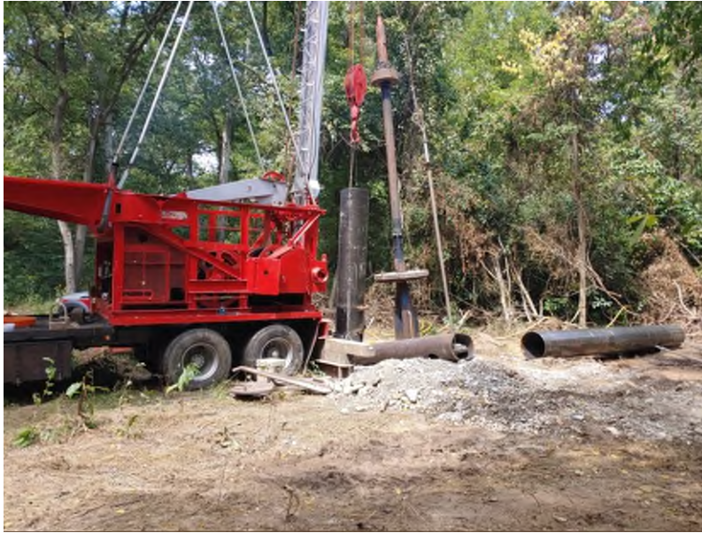
Figure 2. Production well MJ-PW3 under construction at the Middletown-Junction property, August 2024.
