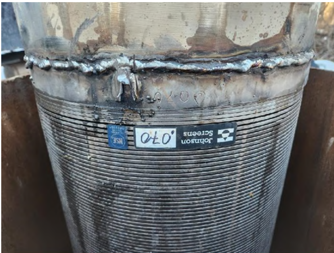
Figure 4. NWS constructing the MJ-PW3 screen and well casing on January 28, 2025.
