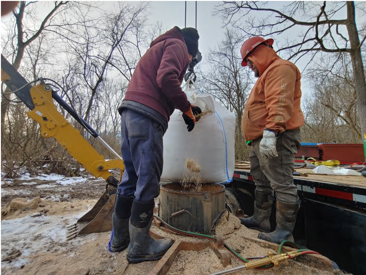
Figure 5. No. 4 Parry sand pack being placed around the well screen, January 30, 2025.
