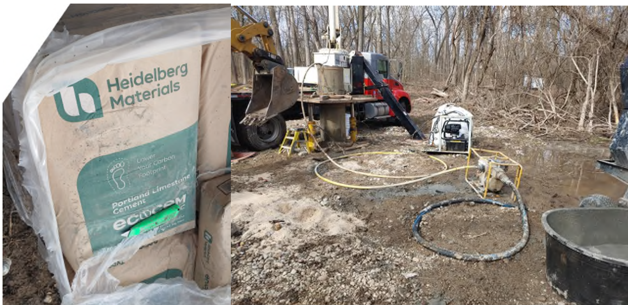
Figure 6. NWS using tremie equipment to seal the annular space of well MJ-PW3 with cement grout, February 4, 2025.
