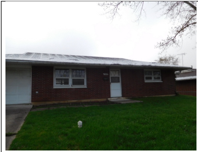
1. Exterior of Structure
