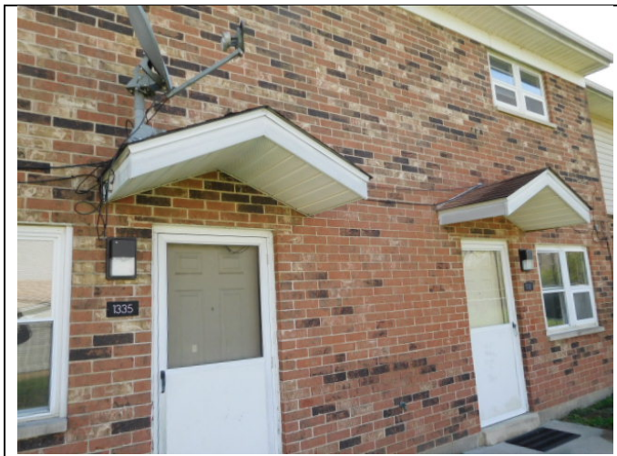
2. Exterior of Structure
