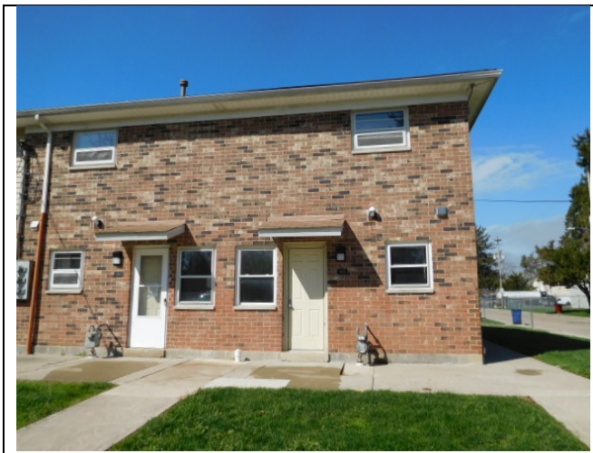
1. Exterior of Structure
