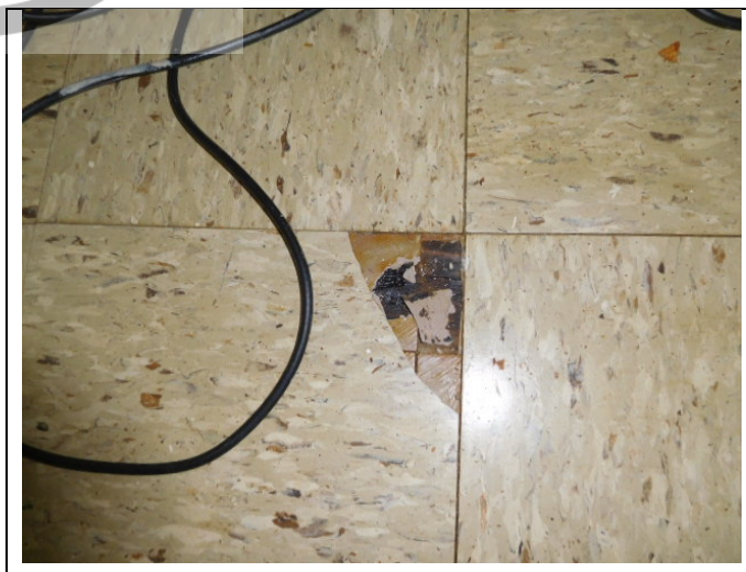
12. 9" Floor Tile beneath 12" Floor Tile
