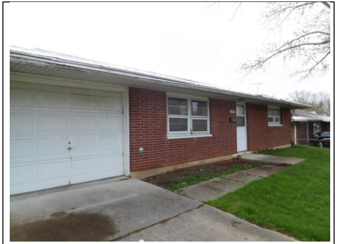
2. Exterior of Structure
