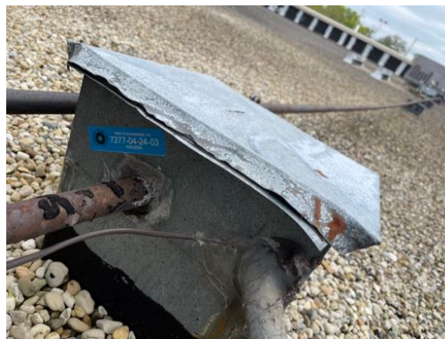
Photo 80- Sample #7277-04-24-03, No Asbestos Detected in Grey Electrical Sealant
