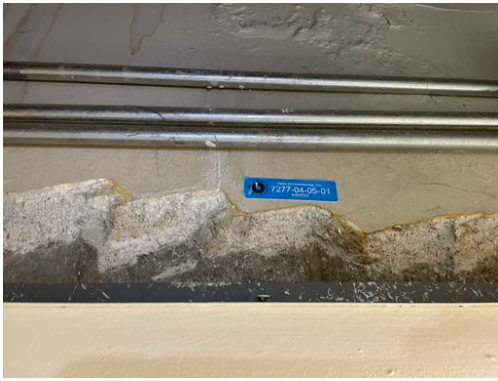
Photo 37- Sample# 7277-04-05-01, No Asbestos Detected in Hard Plaster and Skim Coat
