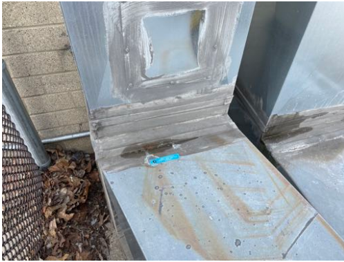
Photo 76- Sample #7277-04-16-16, No Asbestos Detected in Grey Duct Sealant
