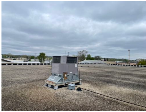
Photo 83- Bituminous Roofing is Assumed to be Category II Nonfriable Asbestos
