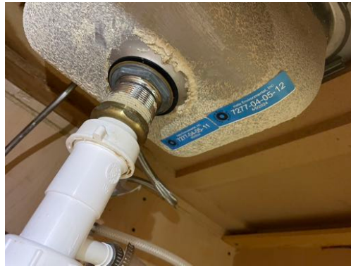
Photo 47- Sample# 7277-04-05-11, No Asbestos Detected in Sink Soundproofing
