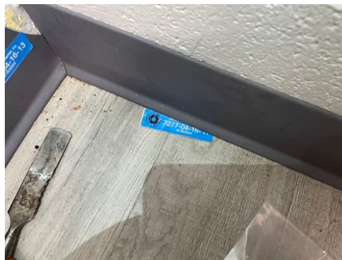
Photo 71- Sample #7277-04-16-11, No Asbestos Detected in Flooring
