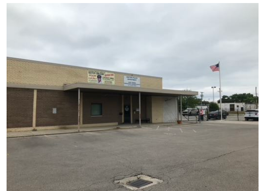
Photo 36- Exterior, South Side, Southeast Area
