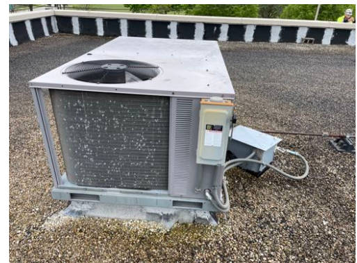
Photo 81- Sample #7277-04-24-04, No Asbestos Detected in Grey Electrical Sealant
