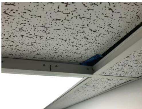
Photo 17- Sample# 7200-05-30-19, No Asbestos Detected in 2' x 4' Ceiling Tile
