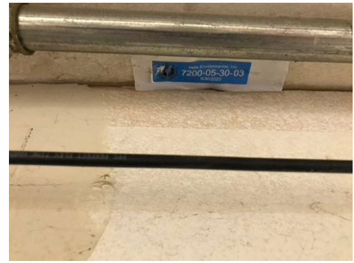
Photo 03- Sample# 7200-05-30-03, No Asbestos in Hard Plaster on Wire Lath
