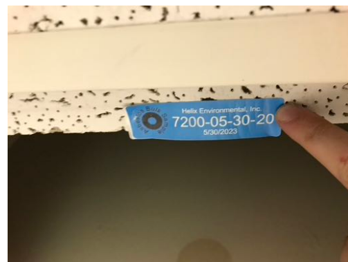
Photo 18- Sample# 7200-05-30-20, No Asbestos Detected in 2' x 4' Ceiling Tile
