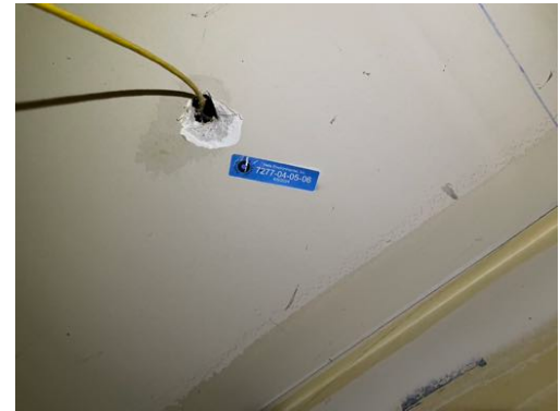
Photo 42- Sample# 7277-04-05-06, No Asbestos Detected in Hard Plaster and Skim Coat
