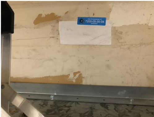
Photo 04- Sample# 7200-05-30-04, No Asbestos in Drywall and Joint Compound
