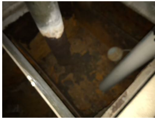
Photo 29- Basement, Northeast Hallway, Former Boiler, No Destructive Inspection Performed
