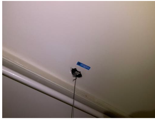
Photo 38- Sample# 7277-04-05-02, No Asbestos Detected in Hard Plaster and Skim Coat
