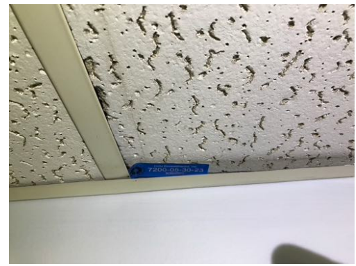
Photo 21- Sample# 7200-05-30-23, No Asbestos Detected in 2' x 4' Ceiling Tile
