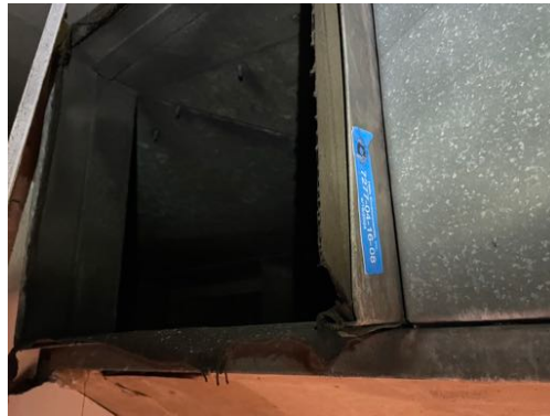
Photo 68- Sample #7277-04-16-08, No Asbestos Detected in Vibration Isolator Cloth
