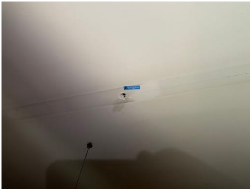
Photo 40- Sample# 7277-04-05-04, No Asbestos Detected in Hard Plaster and Skim Coat
