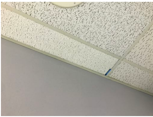
Photo 19- Sample# 7200-05-30-21, No Asbestos Detected in 2' x 4' Ceiling Tile
