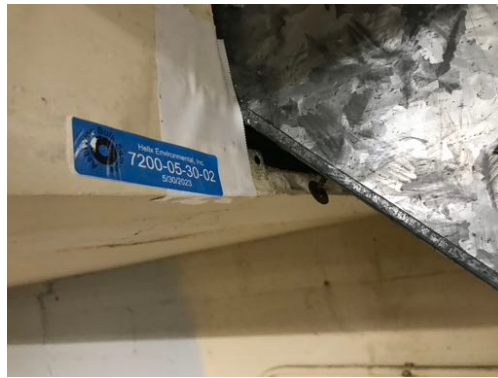
Photo 02- Sample# 7200-05-30-02, No Asbestos in Drywall and Joint Compound
