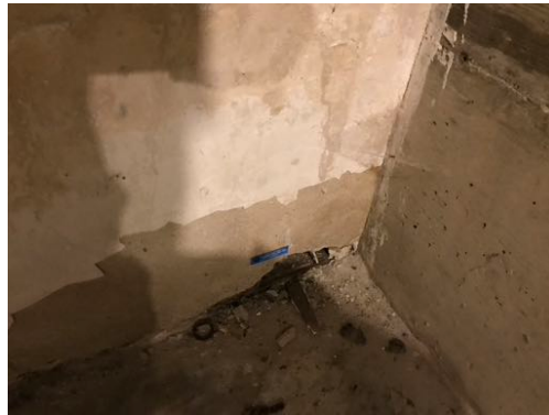
Photo 05- Sample# 7200-05-30-05, No Asbestos in Hard Plaster on Gypsum Lath
