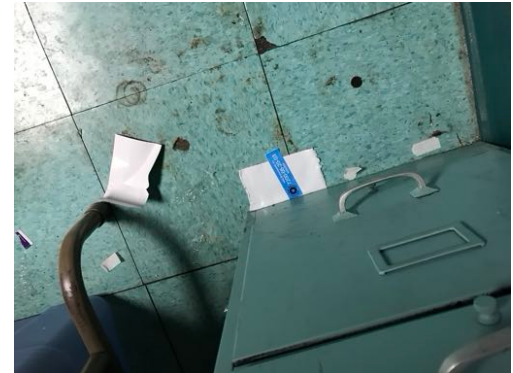
Photo 24- Sample# 7200-06-20-03, No Asbestos Detected in 12"x12" Aqua Floor Tile or Black Mastic, Asbestos Floor Tile Beneath
