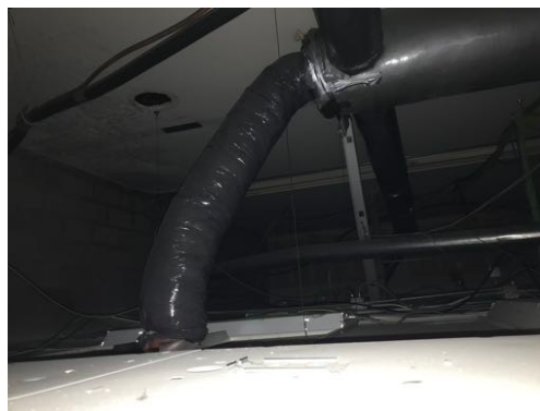
Photo 35- 1st Floor, East Office Area, Hard Plaster on Wire Lath above Ceiling Tile Throughout, No Access to Attic
