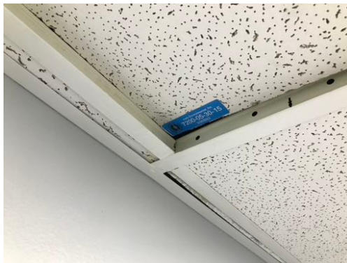
Photo 14- Sample# 7200-05-30-15, No Asbestos Detected in 2' x 4' Ceiling Tile
