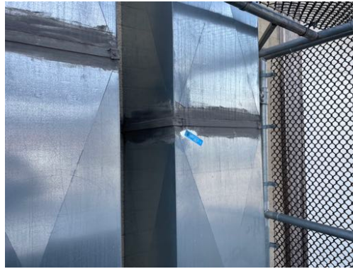
Photo 77- Sample #7277-04-16-17, No Asbestos Detected in Grey Duct Sealant
