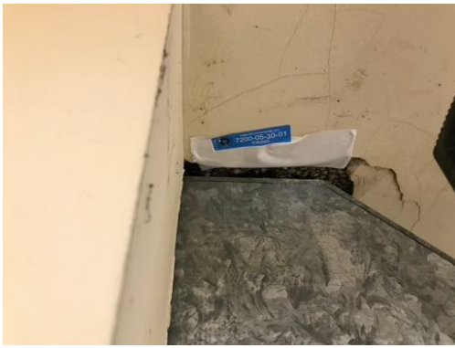
Photo 01- Sample# 7200-05-30-01, No Asbestos in Hard Plaster on Wire Lath
